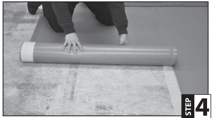
**Step 4:** Roll out the next roll of ComboFoam® in the same manner, making sure that the foam seams are butted together. Be sure to overlap only the moisture barrier lip and not the foam pad.
