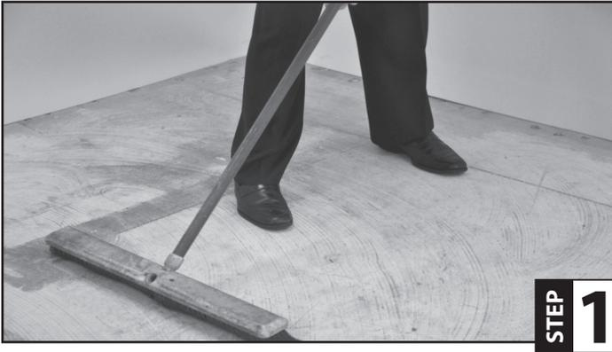
**Step 1:** Make sure the subfloor is structurally sound, level and is free of dust and debris. The deflection cannot exceed  $L/360$  of the span under intended live and dead loads. Check for protruding nails and/or defects in the subfloor. If installing over concrete, the concrete must be dry with moisture emission rates that do not exceed 3lbs. per 1000 square feet per 24 hours as measured by the Anhydrous Calcium Chloride Test.
