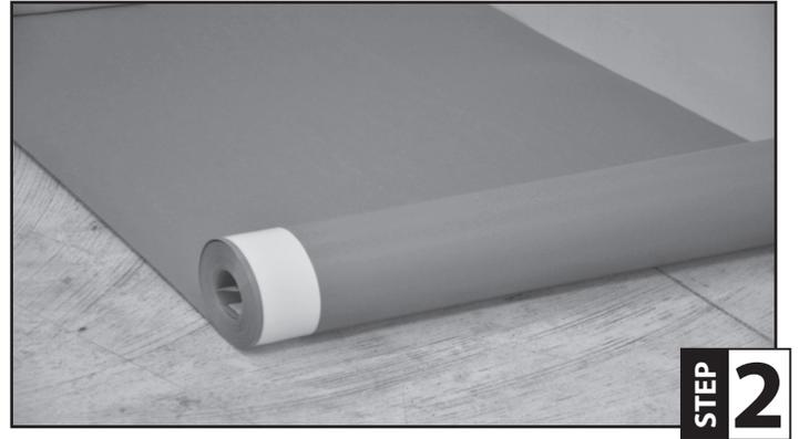
**Step 2:** Start in a corner with tape strip side next to wall and overlapping film toward the open room. Install the ComboFoam® (film side down) parallel to the wall in the opposite direction as you plan to install the flooring planks. When installing the ComboFoam, leave at least 2" going up the wall.
